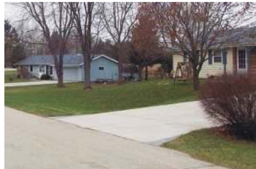
Illegal: concrete extends to edge of public road
