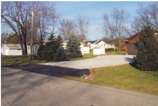
Correct: Blacktop in public road right-of-way
